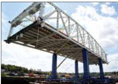
Incremental bridge lifting
