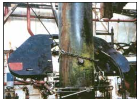
▼ Decommissioning job with band saw.
