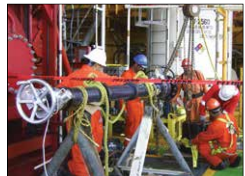
▼ CHT2000 hot tapping offshore application.
